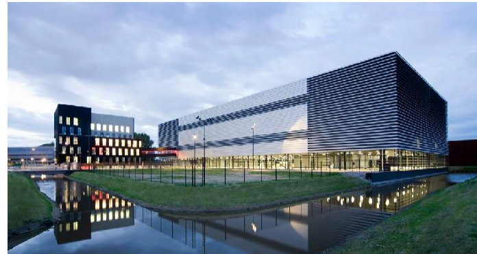
Xtream Server AM3 IBX data center exterior
